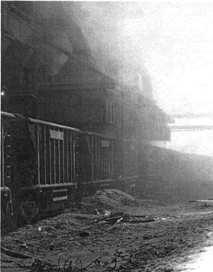
Figure 2. Loading coke onto rail quench cars.
