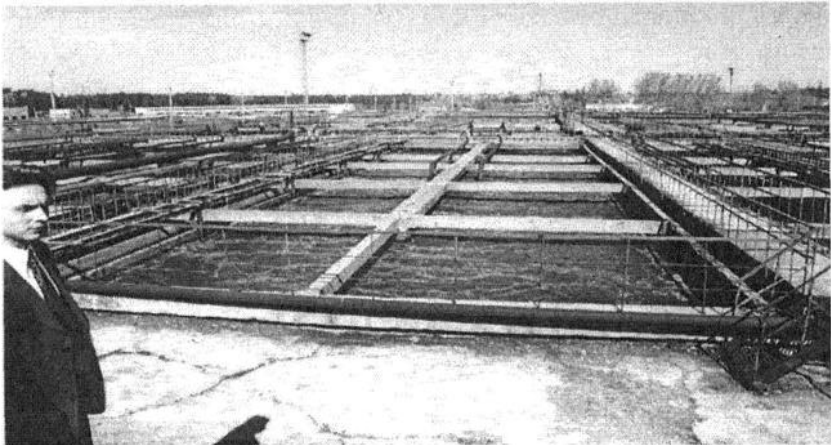
Figure 12. Rectangular settling basins in operation.
